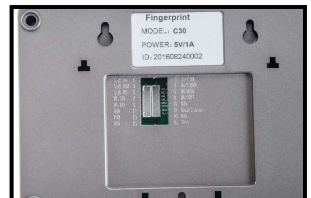
Completed Access Control Connection
